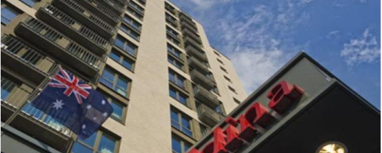
Adina Apartment Hotel Frankfurt Neu Oper (134 rooms) Refurbishment from 3Q 2025
