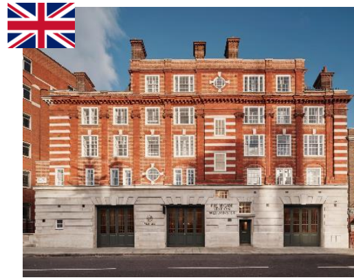
Westminster Fire Station Residential
